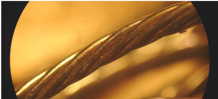
Figure 51 Surface corrosion as a result of carbide precipitation in the area of a welded wire.
