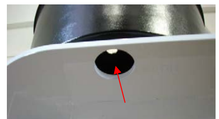
Align the RHGSE cut out with the drainage hole in the tub as shown.
