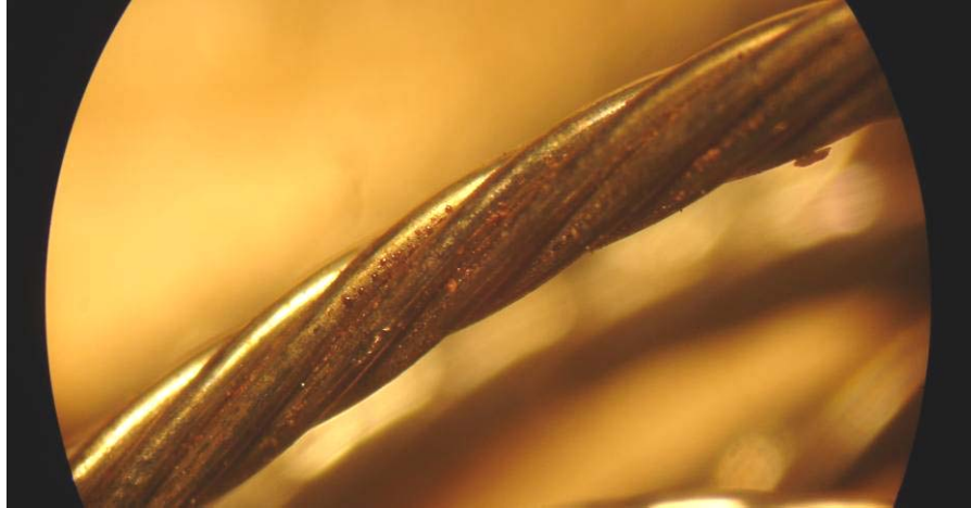
Surface corrosion as a result of carbide precipitation in the area of a welded wire
